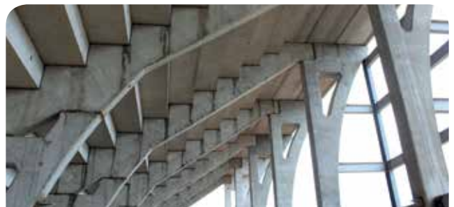
The main contractor started with the brick works at the front of the grand stand to accelerate the works while Corestruc started placing the raking columns
